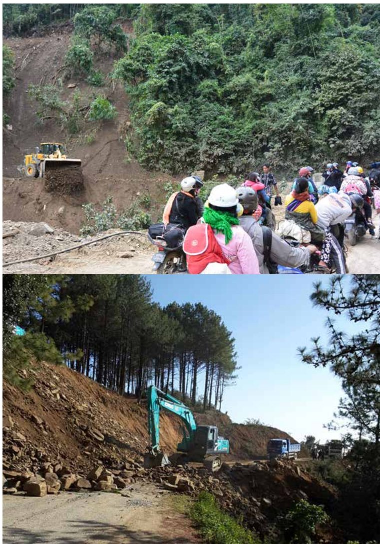
FIGURE 15: Road construction and mobility
