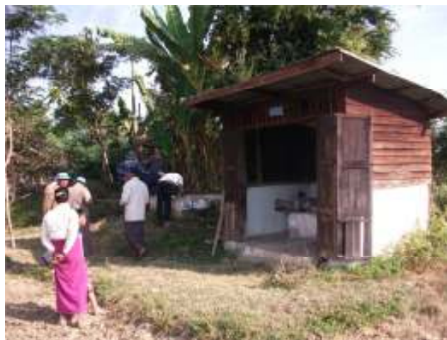
Figure A3.2. Pump house for community irrigation well 4/1 (the stilling tank before distribution is evident to the left of the image)
